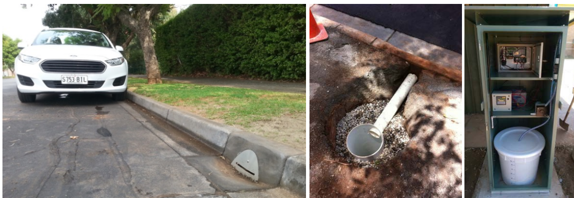
Figure 5. Over 180 TREENET Inlets built into the kerb (left) direct stormwater into leaky wells in the street verge (centre), to provide passive irrigation to street trees and reduce and delay flows reaching the monitoring equipment at the catchment outflow (right).
