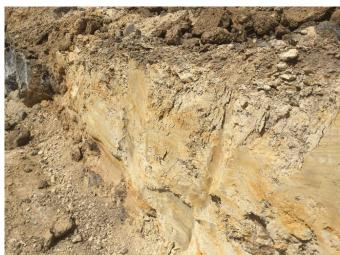
**Figures 1a and 1b.** Dense clay subsoils excavated for tree pits. Note the smearing of the clay (right) by the excavator bucket.
