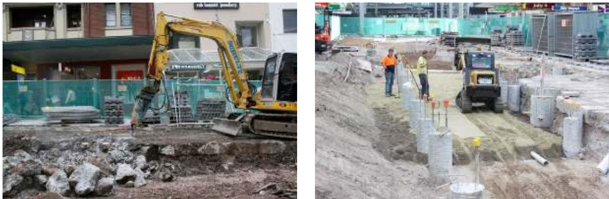
Figure 3. Concrete and compacted rubble materials were removed from the Chatswood site (left) prior to installing quality soil blends in contiguous tree trenches (right)(Images: Arterra, R Smart)
