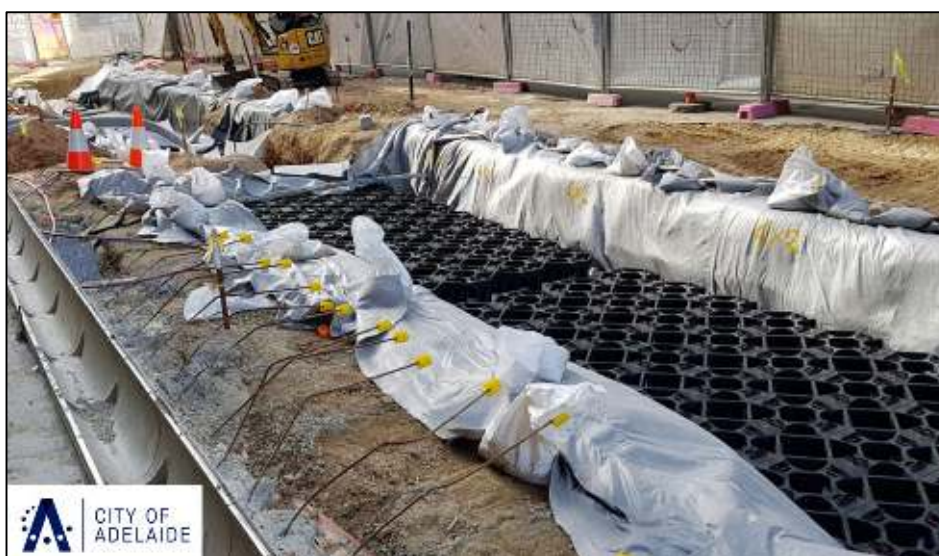
Figure 6. Structural cells were used to support pavements in tree root zones in Bank Street, Adelaide. (image: City of Adelaide)
