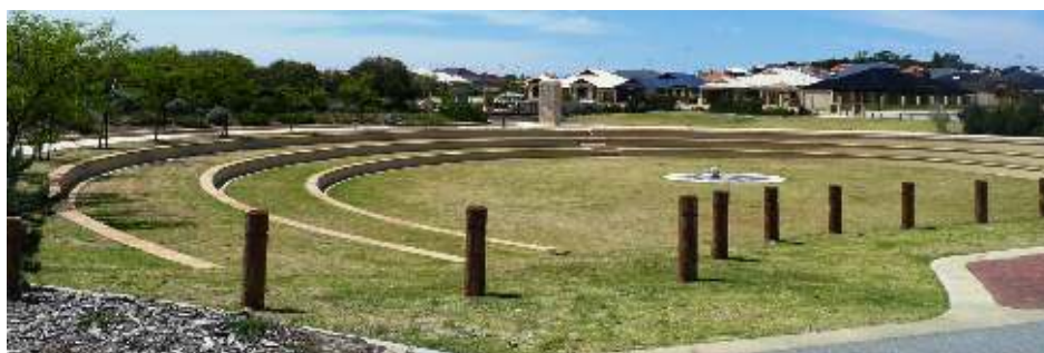
Figure 2. This area provides social and recreational benefits and can manage stormwater from a major rainfall event, with floodwaters draining into underground cells in 24 hours, so it can be available for recreation again quickly.
